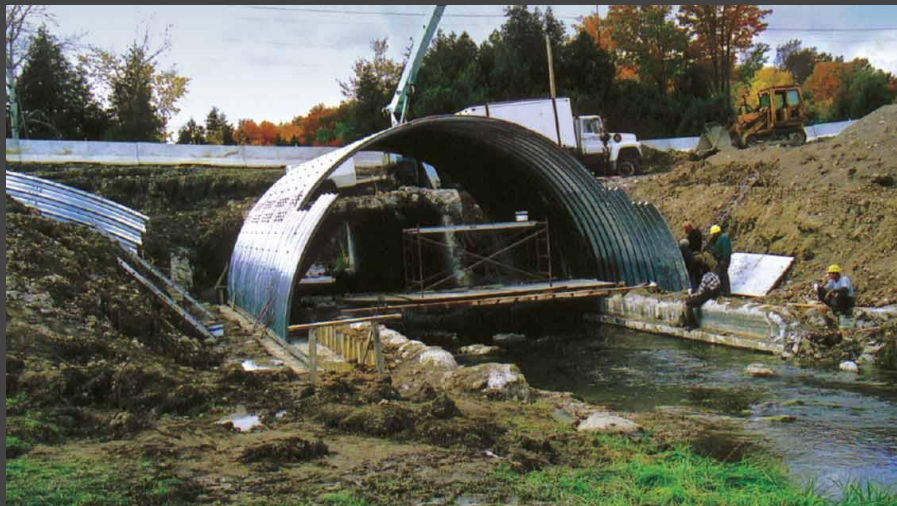
"Bridge-Plate Replaced Distressed Bridge While Keeping Highway Open." Armtec . Armtec, n.d. Web. 07 Dec. 2016.
